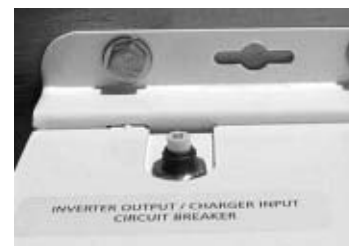
Circuit Breaker Reset
